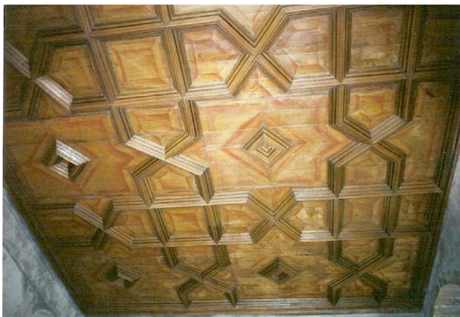
Fig. 3. Kinneil House, Bo'ness, coffered oak ceiling executed for Regent Arran, c. 1542-56, the pattern copies a design from Serlio. Photo author.
